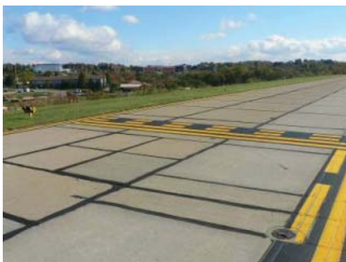
KPIT Taxiway E enhanced hold-short line and wigwag warning lights
