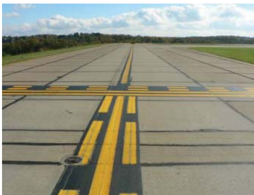
KPIT's Taxiway E hold-short line for Runway 28C.
